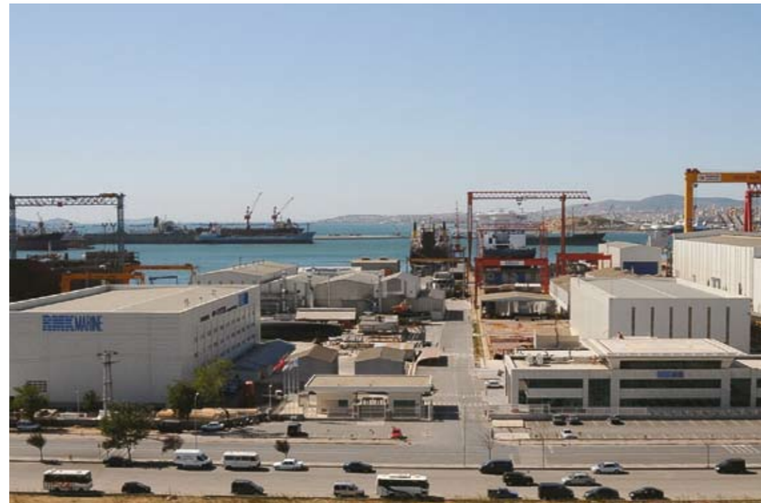
Below: A huge 95,000m 2 facility at Tuzla, just 45km from Istanbul, hosts all three divisions of the RMK Marine operation
